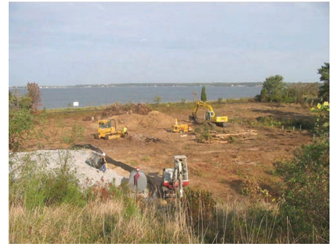
Environmental restoration work in 2007 to remove lead-contaminated soil from a closed rifle range (Operable Unit 2-Area E) at NAS Patuxent River.
